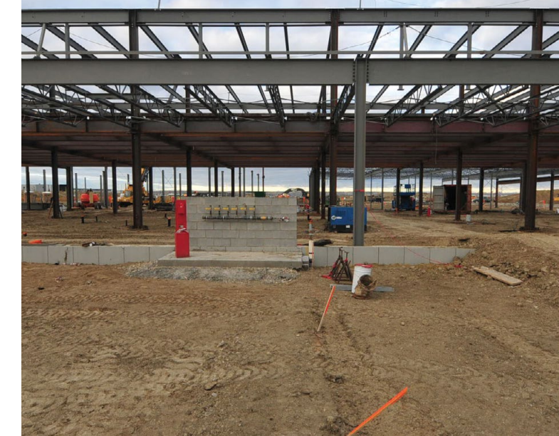
Construction progression showing structural steel shell of the new building.
