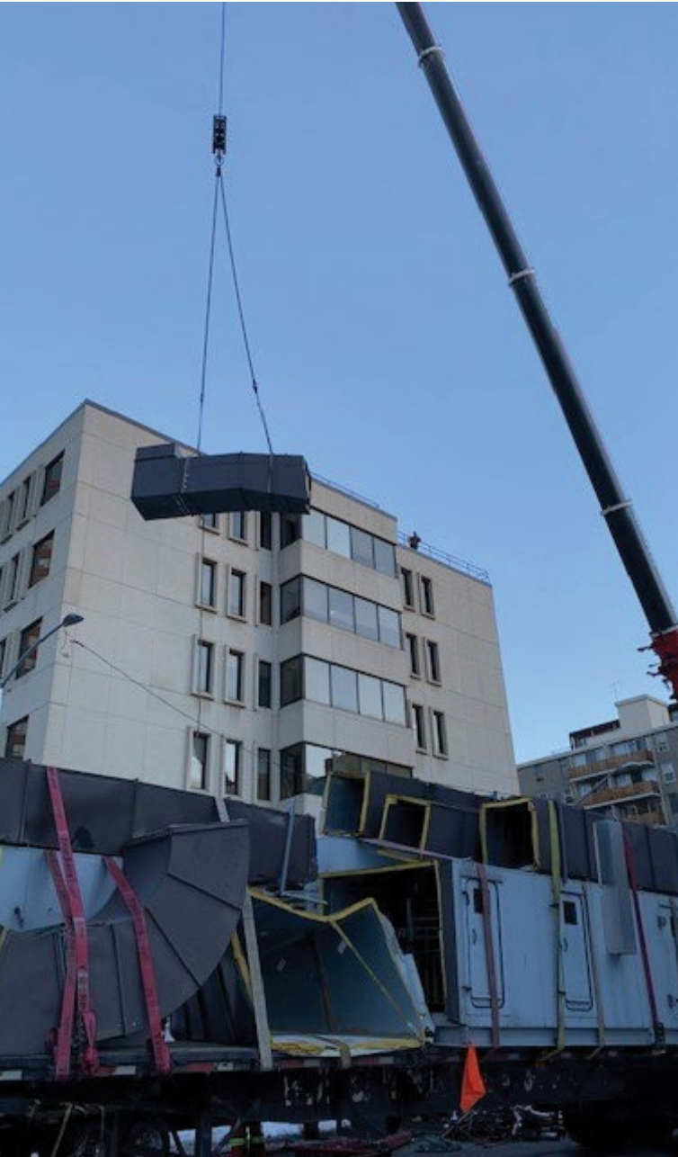
Decommissioning of the fifth and sixth floor laboratory air handling units from 737 - 13th Avenue SW.
