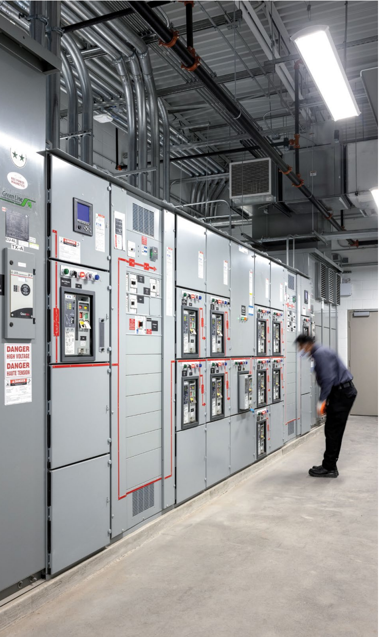
Electrical switchgear controlling the primary power and generator backup to the building. The large conduits feeding the electrical switchgear panels were digitally modelled, fabricated off site and installed ready for use.
